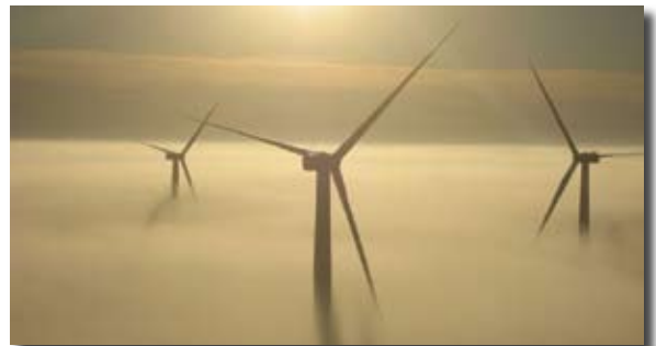
Photos courtesy of Wind Capital Group
